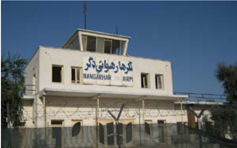
Jalalabad Airport control tower
