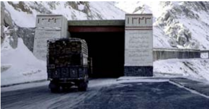
Entrance to the Salang Tunnel
